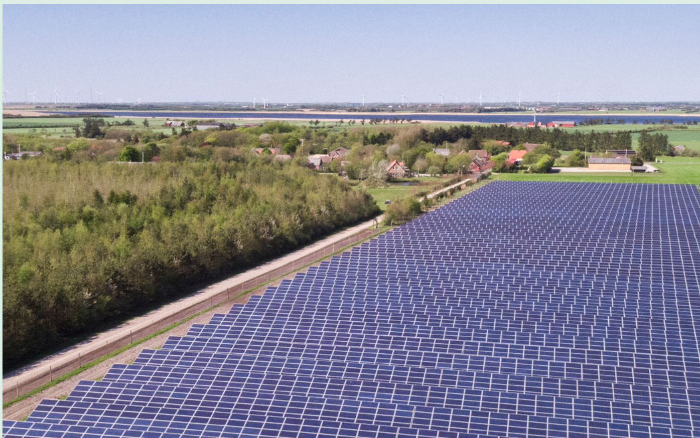
NRGi Solcellepark Nees
